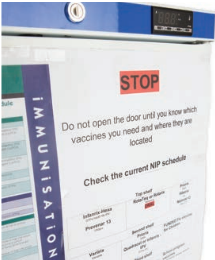
Figure 1: Solid-door purpose-built vaccine refrigerator with map
